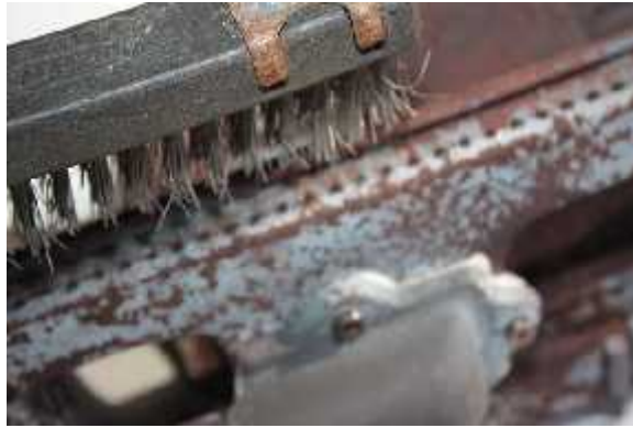
Burner brushed down and partially cleaned.
