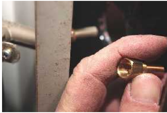
The orifice from the right valve is under another valve.
