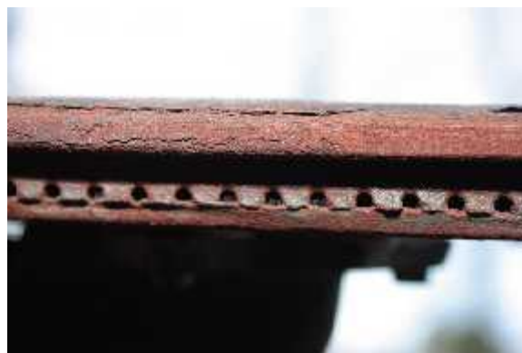
Blow gas ports with compressed air.
