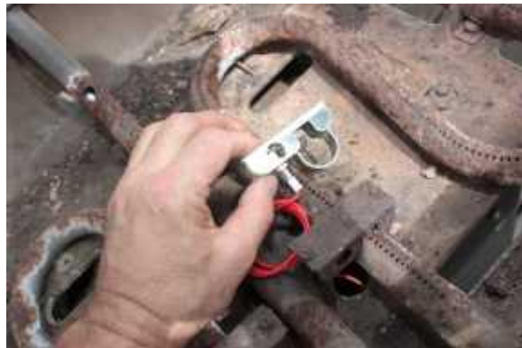
Replace the electrode-collector on the old burner (which is still useable).
